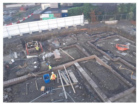
View North – Liftshaf walls and blockwork rising walls being constructed
