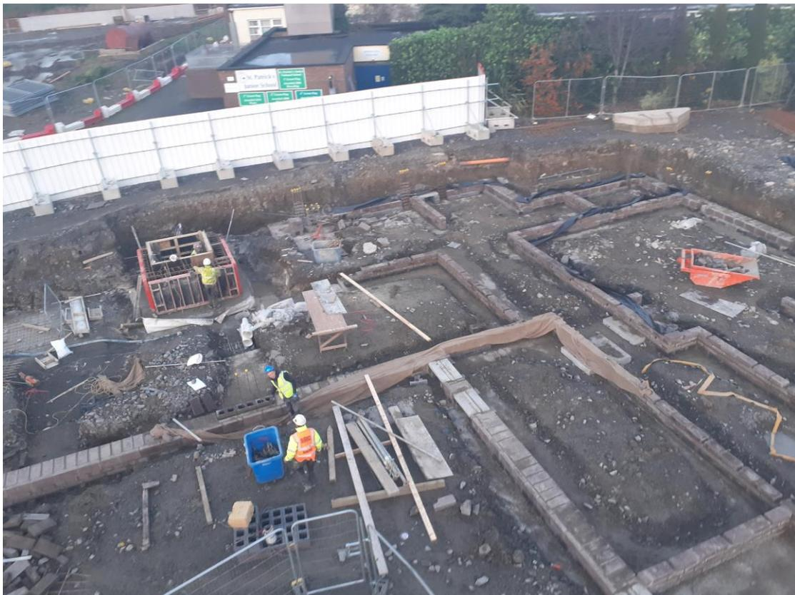
View North – Liftshaf walls and blockwork rising walls being constructed
